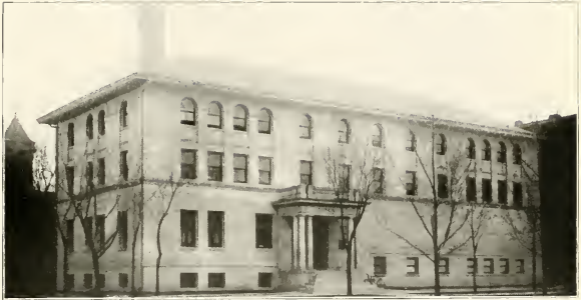
Y. M. C. A. BUILDING, HASTINGS
